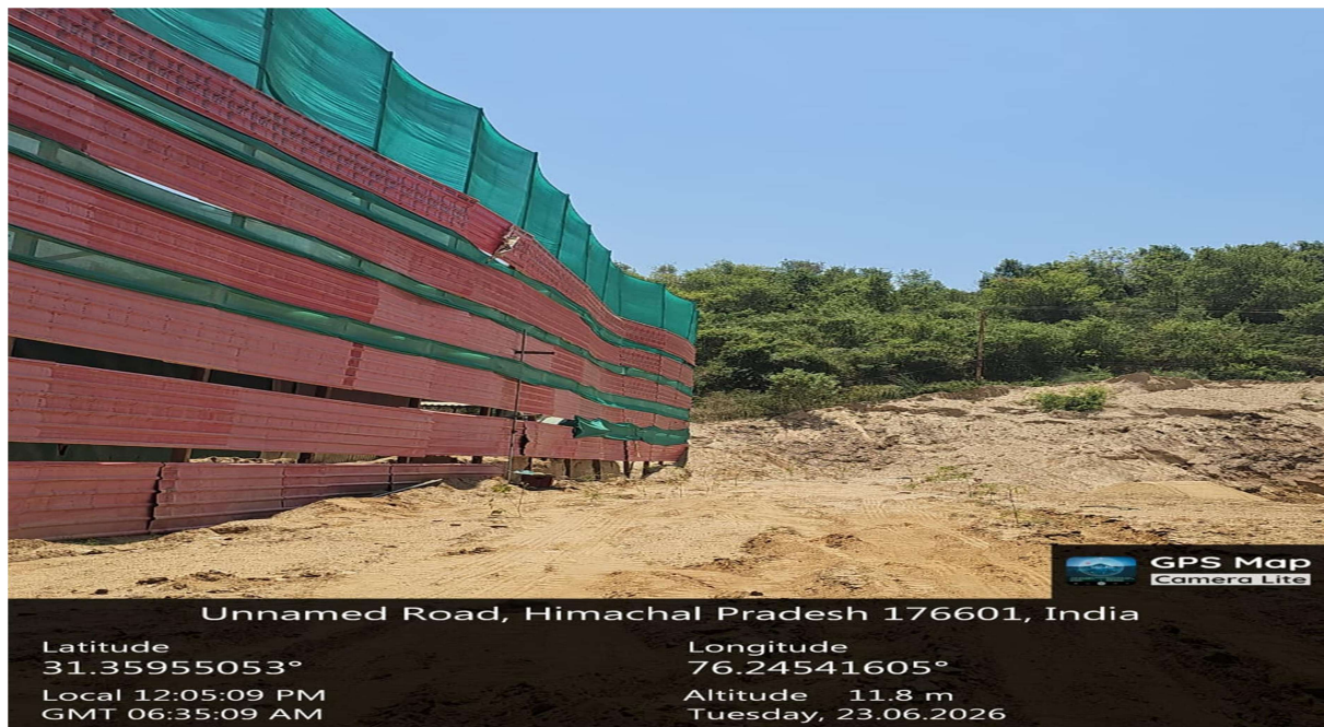
Wind Breaking wall
